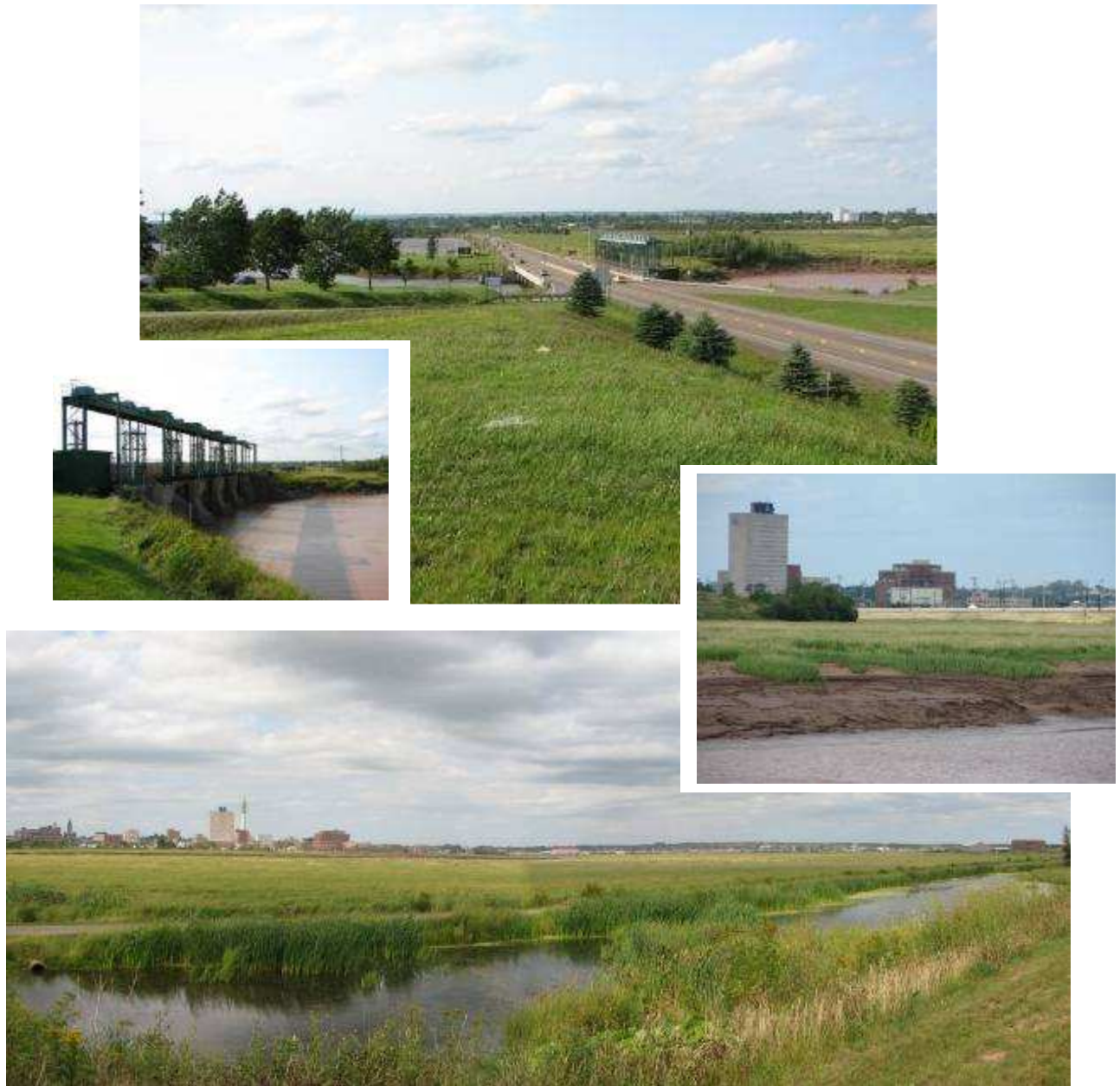
The road causeway over the R. Pedicodiac at Moncton has led to significant build up of mud flats & salt marsh.
